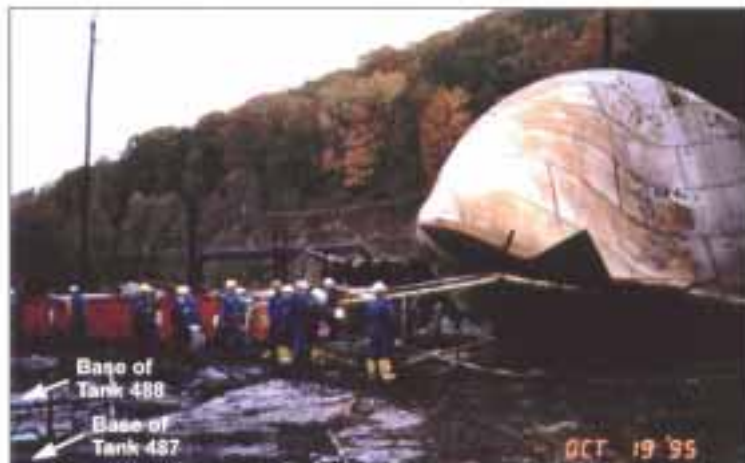
B. Dips in ground showing the original site of tanks 487 & 488. Tank 487 in background.
