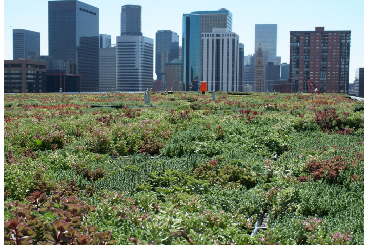
Green roof absorbs heat and CO 2 and reduces stormwater runoff.
