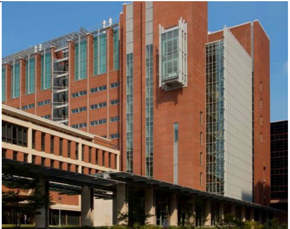
The new UM Dental School building in Baltimore is a state-of-the-art facility treating the dental needs of homeless Veterans.
