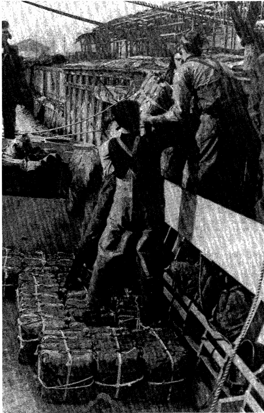
As the evacuation of Hungnam nears completion, explosives are placed on a pier
