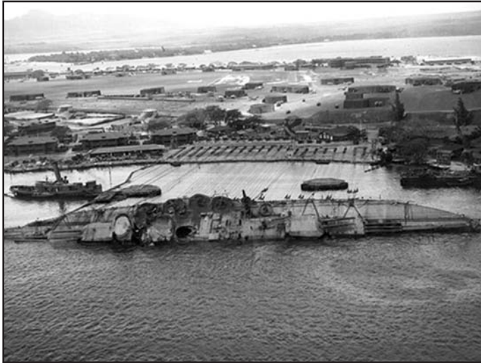
Figure 77. Twenty-one winches right the USS Oklahoma .
