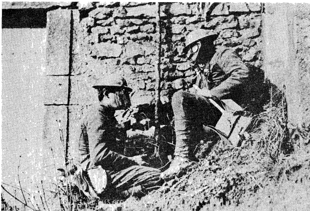
Men detailed to use Ayrton or British trench fans after gas attack, 1918.
