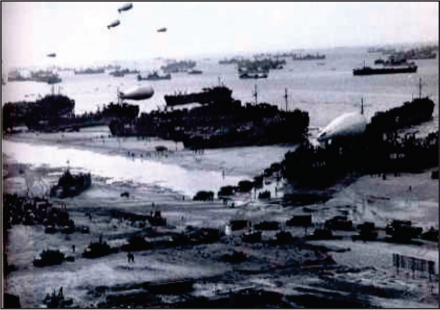
End of the day at Omaha Beach. American equipment coming ashore in staggering numbers. (U.S. Coast Guard)
