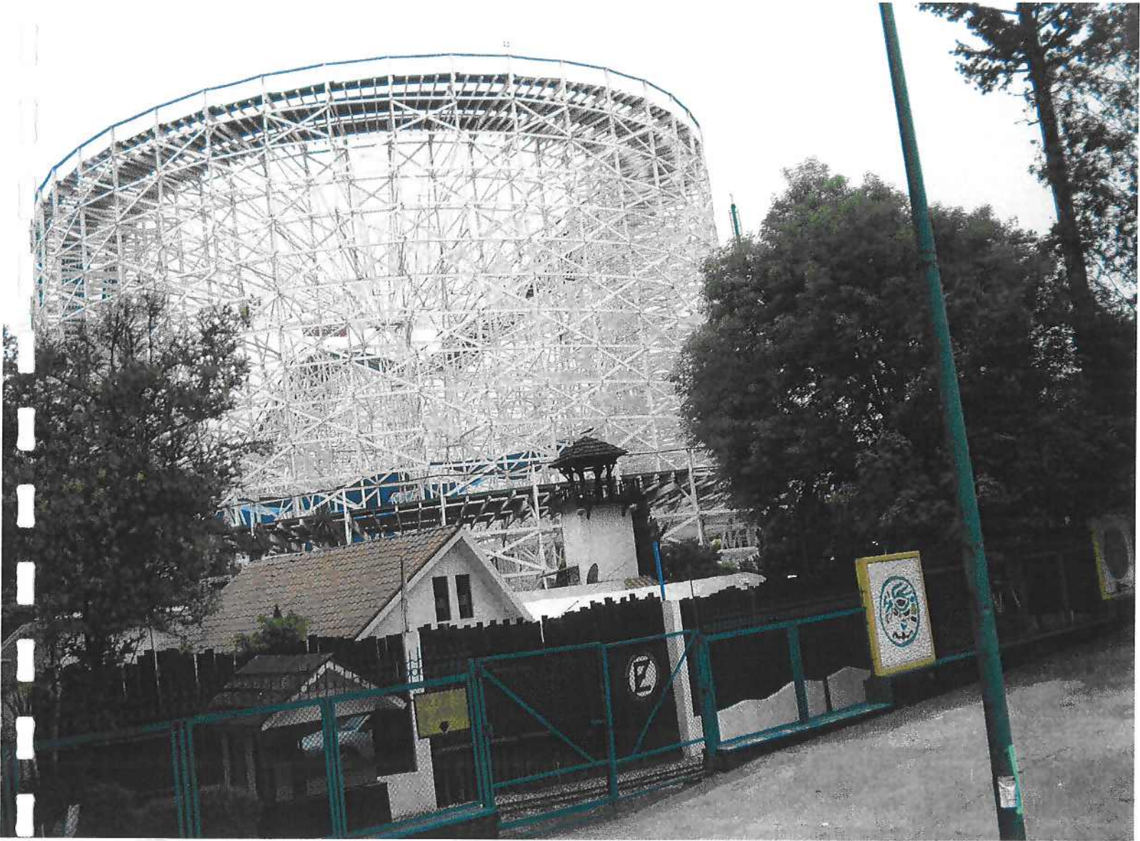
North Side Of Rollercoaster (Beluga Pool Located Under Blue Canopy)
