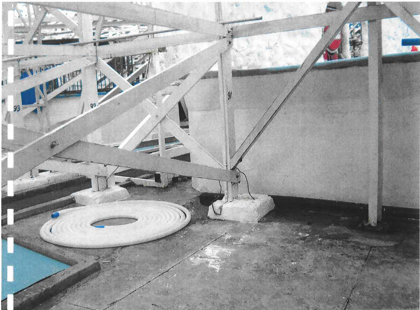
Rollercoaster Supports Embedded In The Concrete Slab Surrounding The Pool
