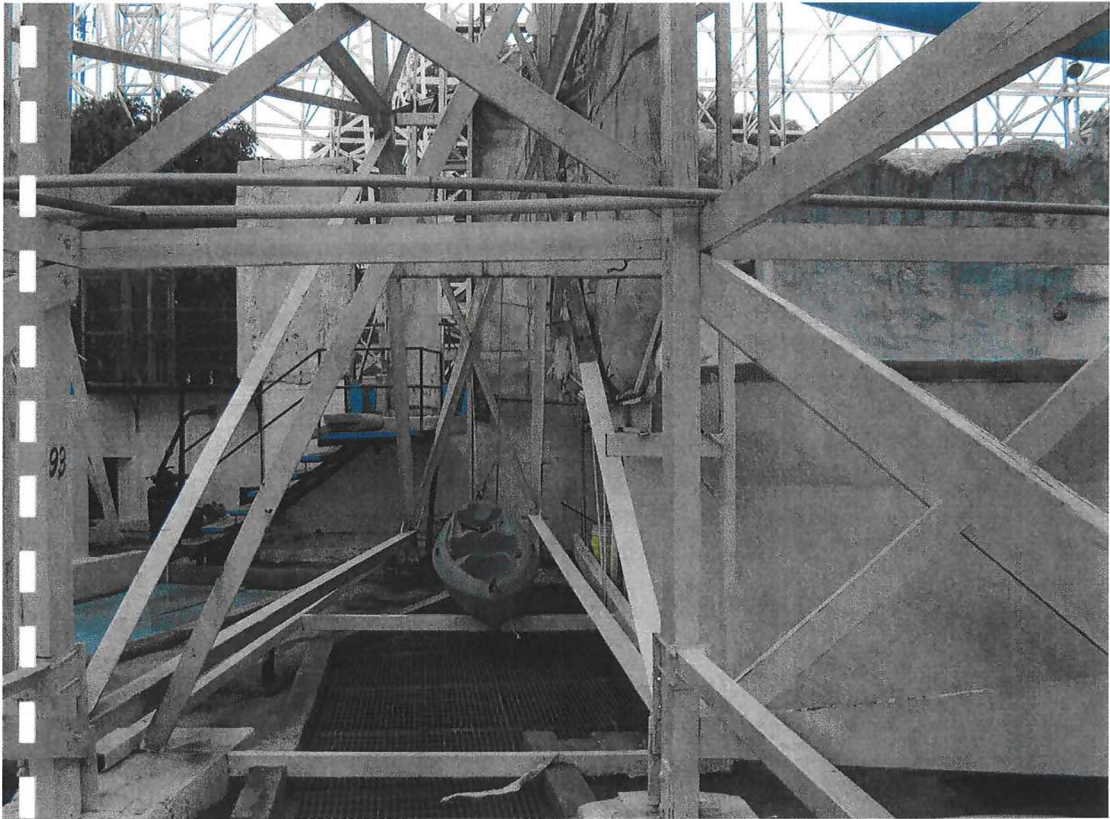
Rollercoaster Supports Embedded In Concrete Slab Surrounding The Pool
