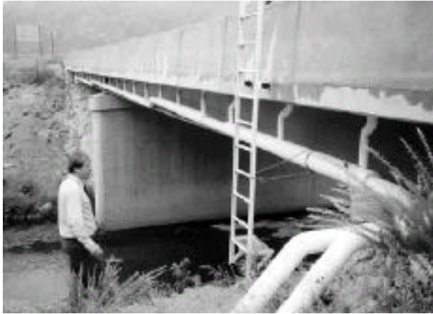
Fig. 4. Left: Heated polypropylene-water solution flows to heat pipes through an 89 mm (3 1/2 in) pipe inside a 152 mm (6 in) manifold on side of bridge. Right: The working fluid is contained within the larger pipe and is vaporized by heat from the furnace-heated liquid pumped through the smaller pipe. The vapor diffuses into the Perkins tube placed horizontally in the deck, gives up its heat of vaporization, and condenses as it is cooled by loss to the deck. The condensate flows back to the reservoir in the large horizontal pipe and is reheated.
