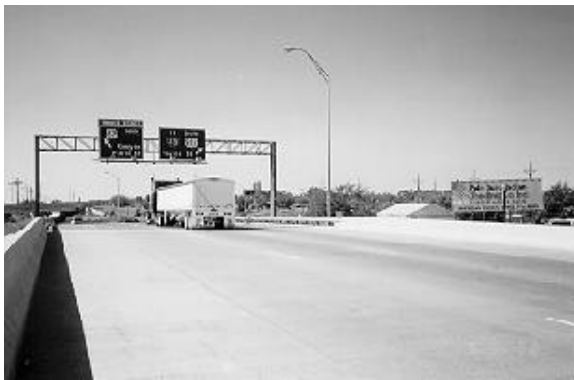
Fig. 1. One of the two two-lane heated bridges on US 287 over N. 15th Ave. in Amarillo.
