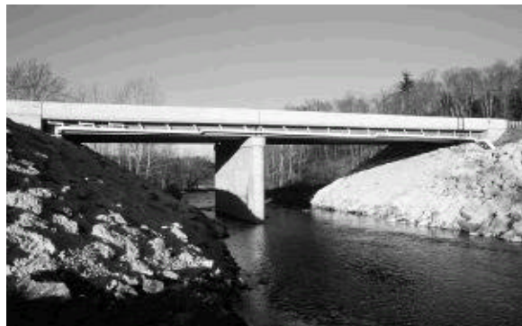
Fig. 1. Two-span bridge is 35.7 m (117 ft) long and 13.4 m (44 ft) wide.
