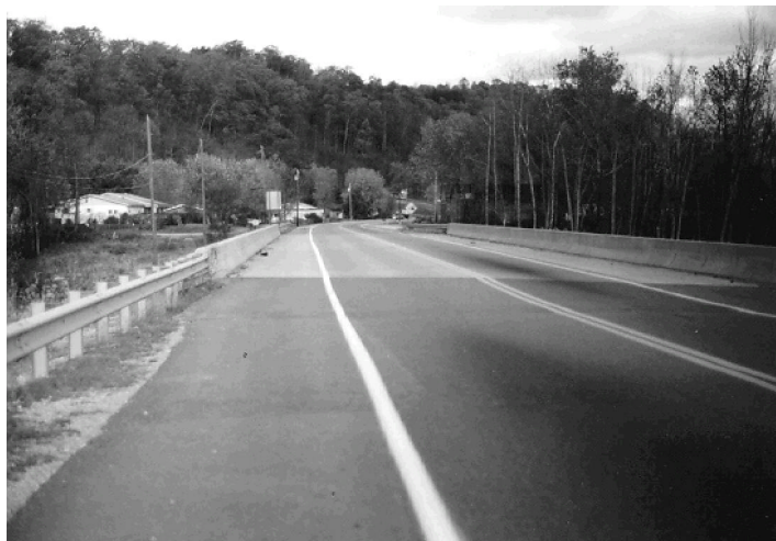
▲ Fig. 2. View of bridge on US 35 over 5&20 Creek. Fig. 3. Meteorological station adjacent to bridge. ➤
