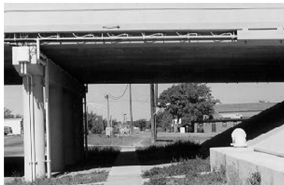
Fig. 2. Manifold conducting heated solution to embedded heating pipes runs alongside of bridge.
