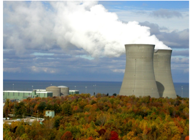
Perry Nuclear Power Plant in North Perry, OH
