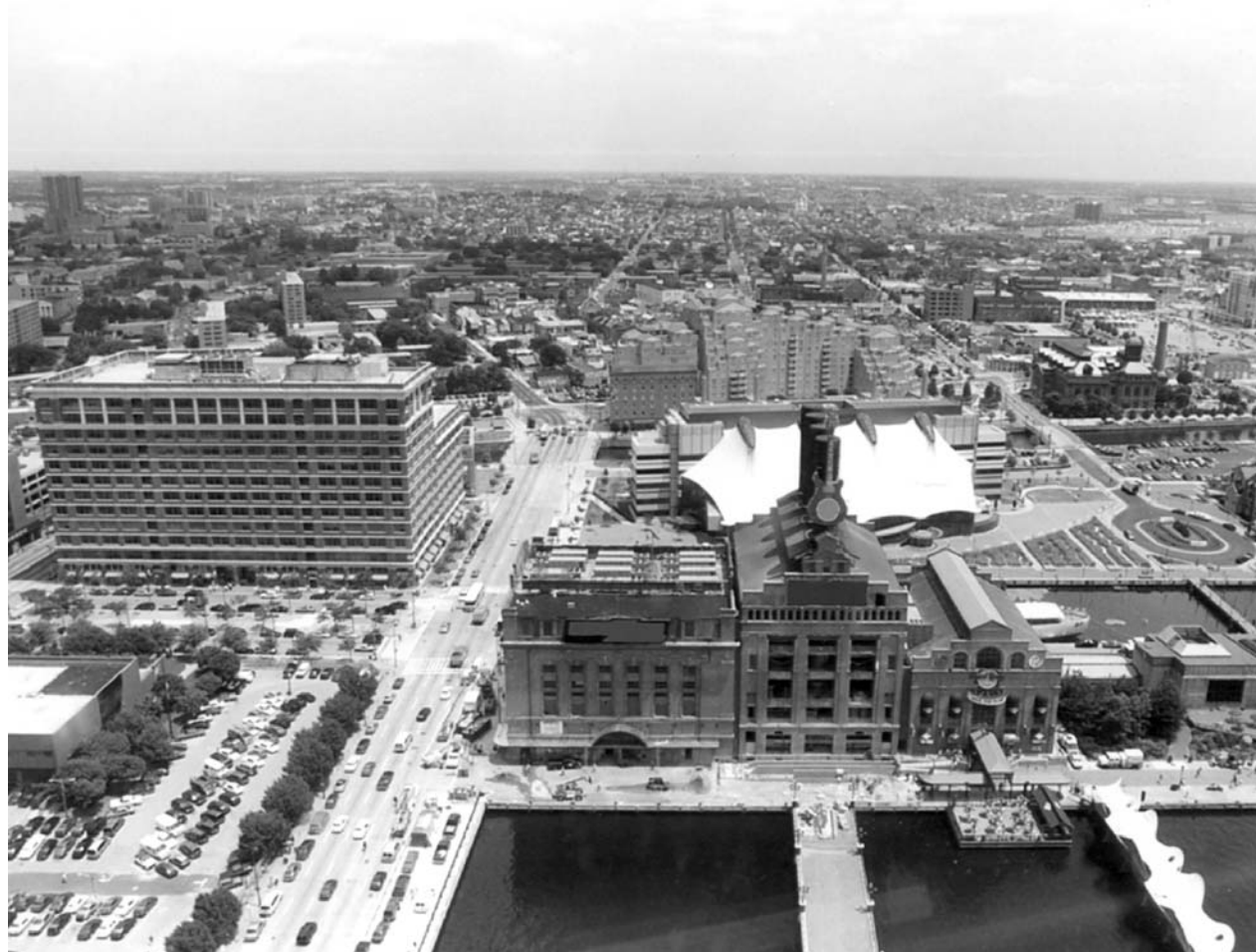
Office buildings, industries, residences, and transport systems, Baltimore, Maryland; east view from the inner harbor. Source: U.S. Department of Energy.
