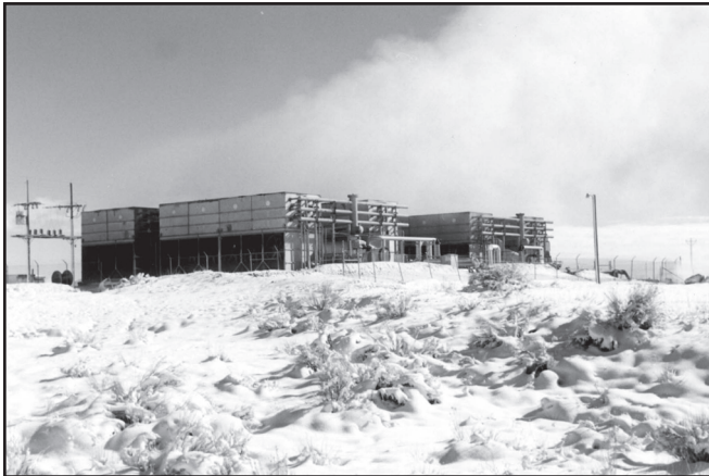
Figure 3. Amedee Geothermal Venture 2-MWe binary plant.
