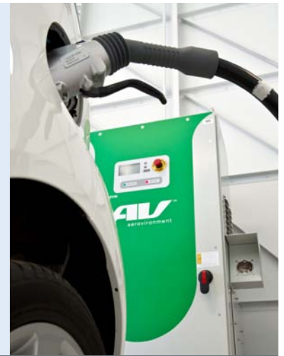
Automotive fast charger enabling 60 miles of range from 20 minutes of charging. Photo by Dennis Schroeder, NREL/PIX 19929
