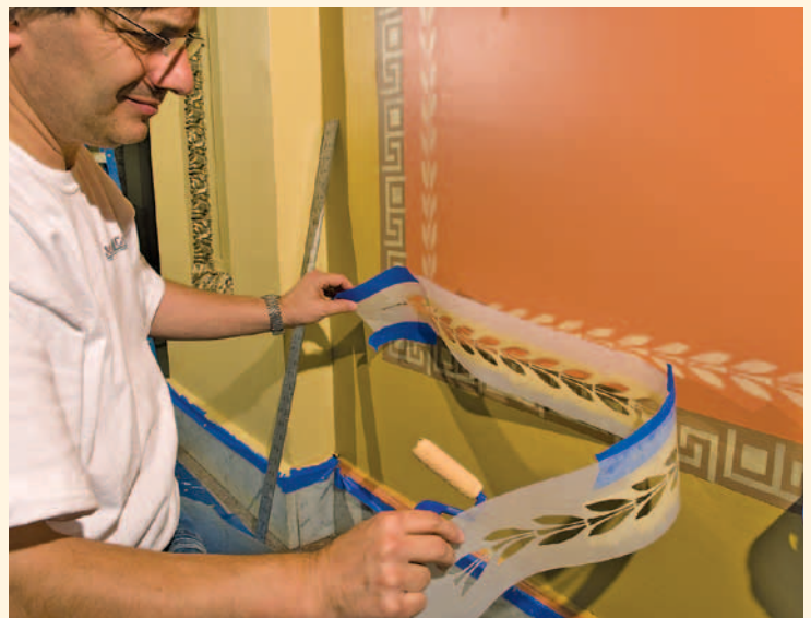
The 1901 leaf border design on a panel in the Capitol's second-floor West Front corridor is recreated by stencil during the FY 2009 conservation and restoration project.
