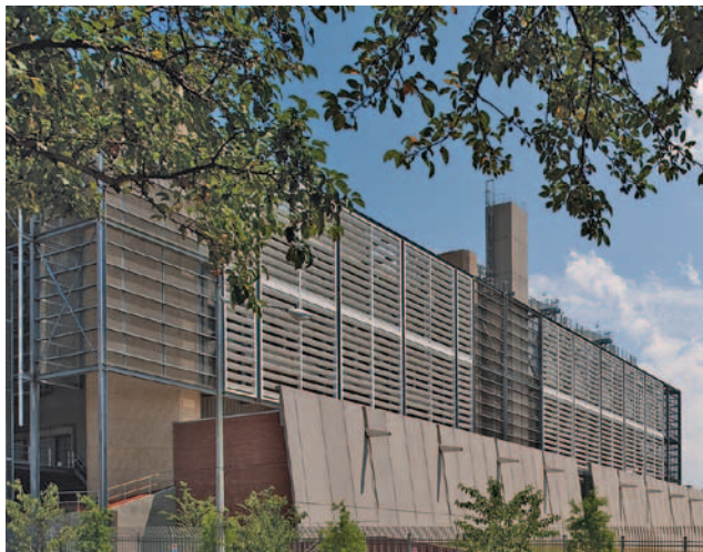
The Capitol Power Plant operates 24 hours per day, 365 days per year, and provides steam for heating and chilled water for cooling the buildings on the Capitol complex.
