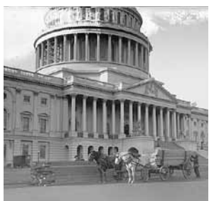
The platform and stands are constructed entirely from scratch for each Inaugural Ceremony. This photograph shows the delivery of lumber to the Capitol for the construction of the 1921 Inauguration stands.
