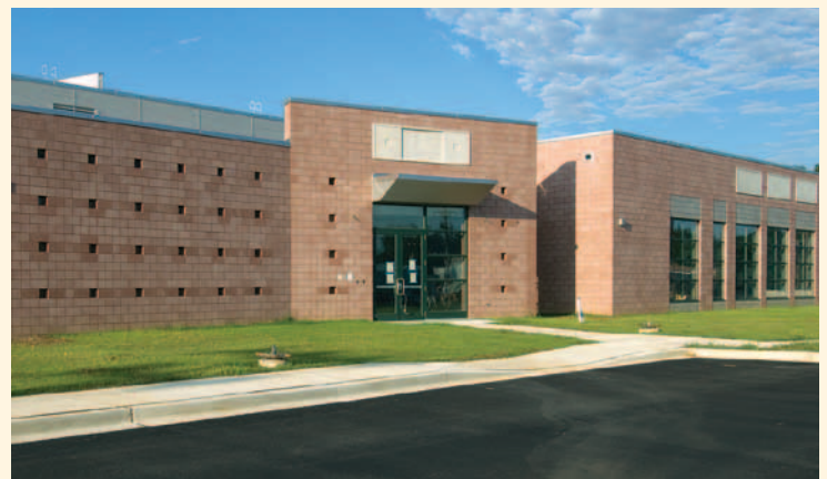
The AOC completed the construction of two state-of-the-art, high-density Book Storage Modules at the Ft. Meade complex in Maryland to support the Library of Congress' preservation capabilities for its special collections.
