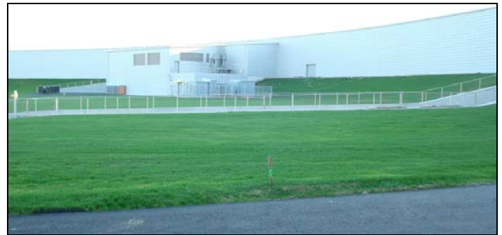
Figure 9. Site restoration completed for interior courtyard.
