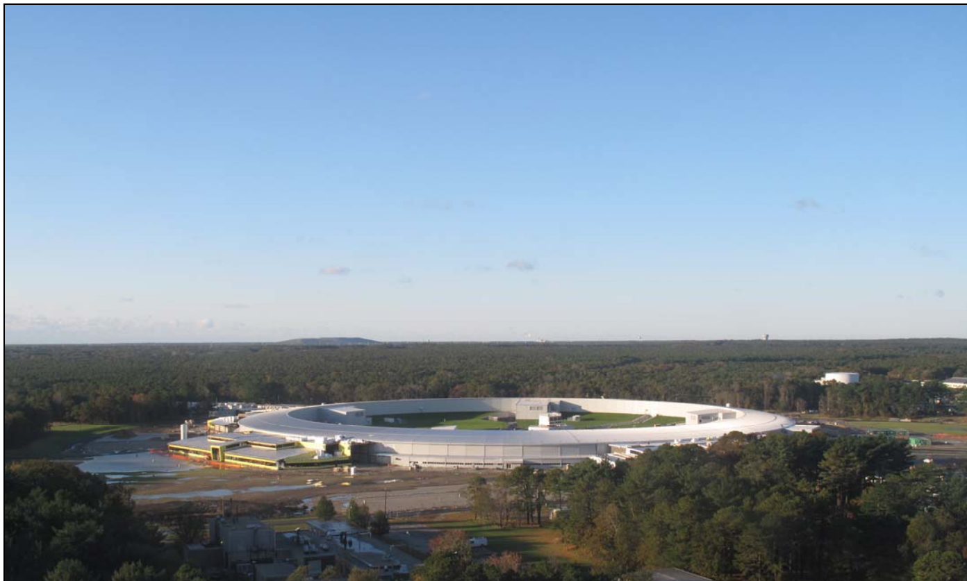
Sunrise after a rainy night in late October. Lab–Office Building (LOB) 2 is nearly enclosed and most LOB activity has shifted to LOB 3, barely visible here.
