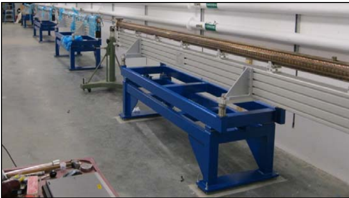
Figure 4. Linac structures in linac tunnel.
