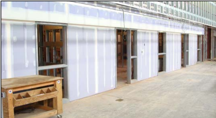
Figure 10. LOB 2 drywall work is underway.
