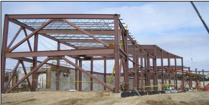
Figure 7: Steel erection for the RF building in early March, near pentant 1.
