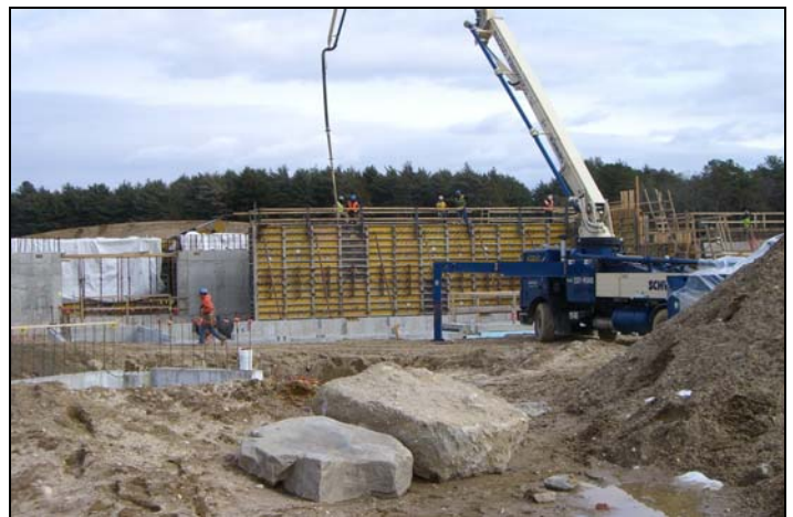
Figure 6: Concrete work for the storage ring tunnel.
