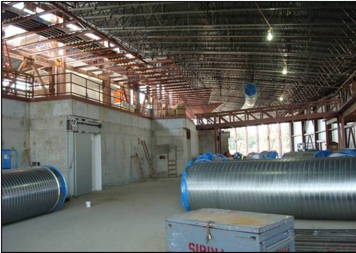
Figure 6. Mechanical-electrical-plumbing (MEP) work underway in pentant 1.
