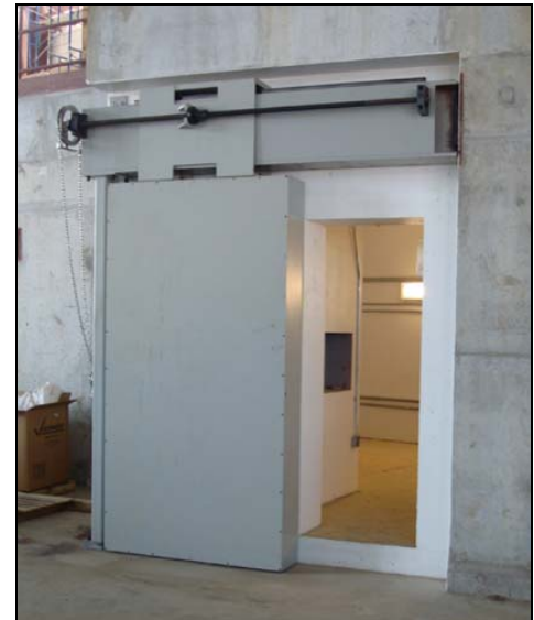
Shield door installation is a portal to the future.
