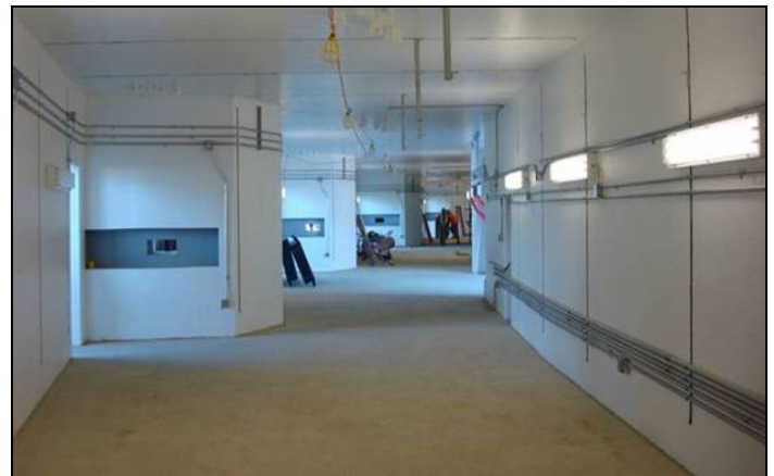
Figure 5. SR tunnel in pentant 1 painted, with conduit and lighting installed.
