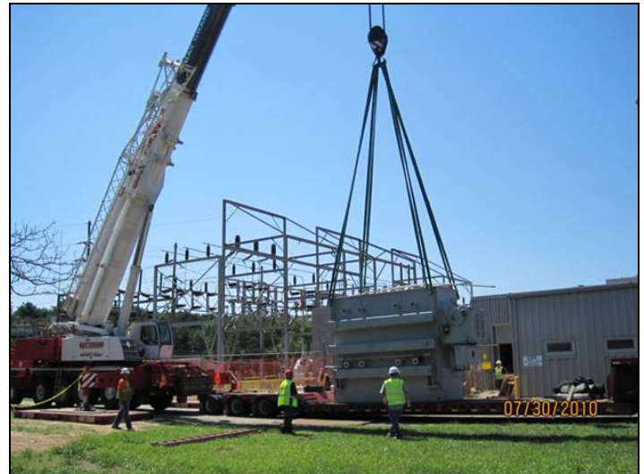
Figure 8. Rigging the 20Mva transformer into the substation on July 30.
