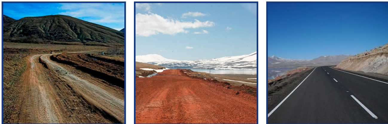
From left to right, the Samtskhe-Javakheti Road before rehabilitation, during construction and once completed.
