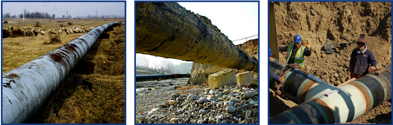
From left to right the gas pipeline repair before and after.
