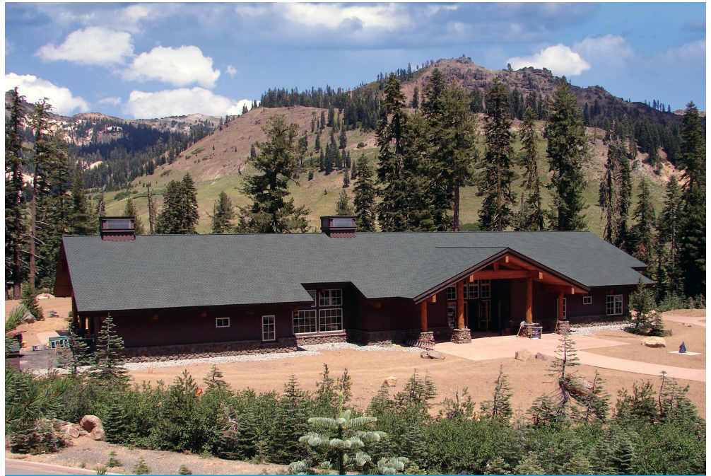
Lassen Volcanic Visitors Center, Mineral, CA. FEMP strives to attract small facilities similar to the Lassen Visitors Center to participate in the ESPC ENABLE program.
