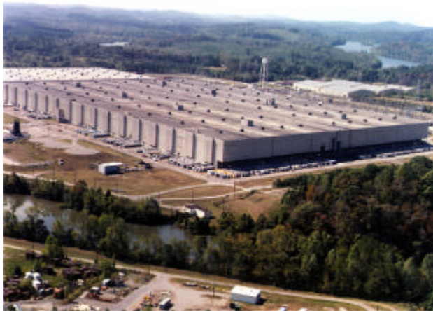
Figure 1. Indoor-PCAT will be within the K33 Building, a two-story building with 33 acres under roof, at the East Tennessee Technology Park.
