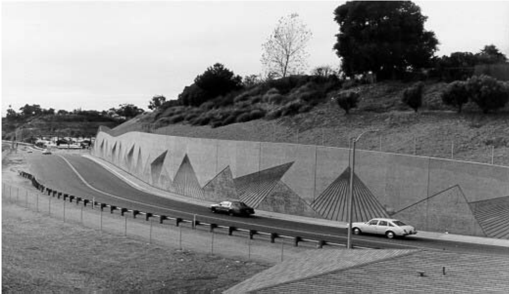
Figure 4.11: Cast-in-Place Facing.
