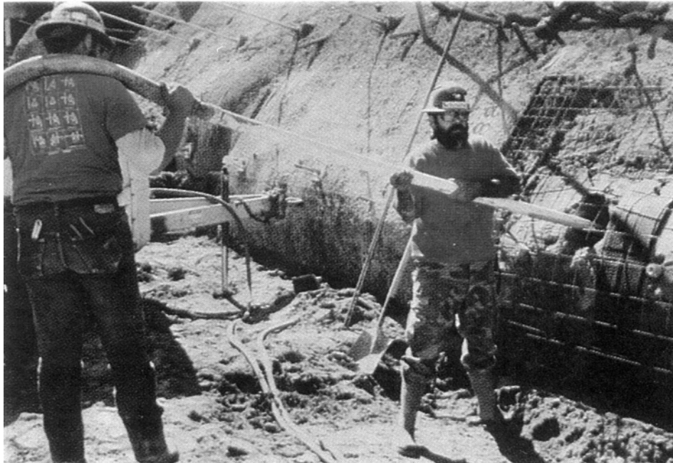
Figure 4.2: Grout Placement (Tremie) through Pipe.
