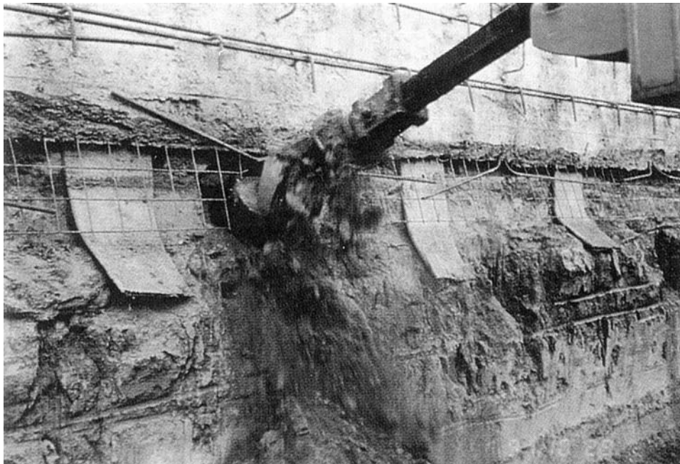
Figure 4.5: Strip Drains under Temporary Shotcrete.
