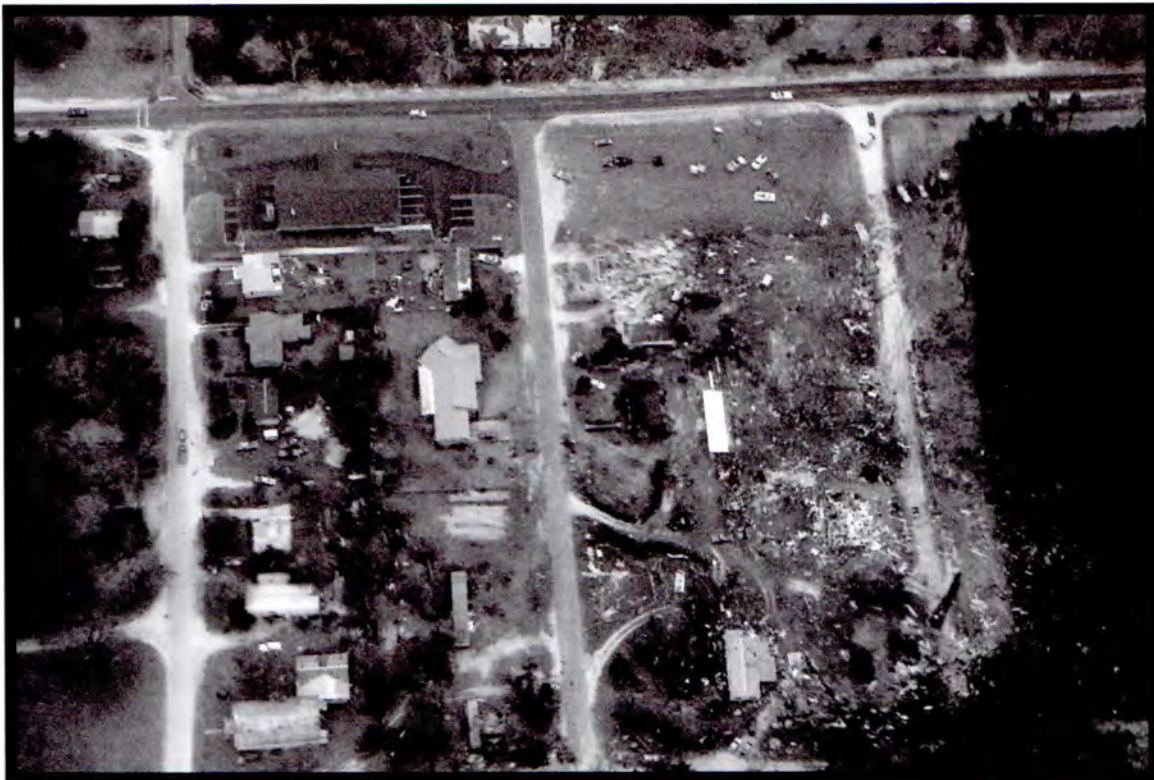
Figure 1-1. Aerial photo of destroyed homes. (Photo courtesy of Brian Smith.)
