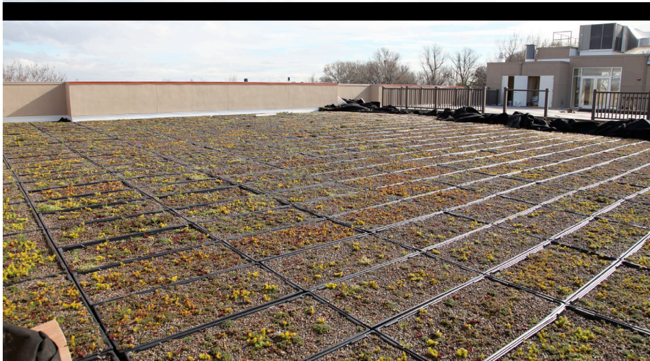
The Philadelphia Housing Authority has begun including green roofs on its new mid-rise senior buildings, like this one at Warnock Village in North Philadelphia. Source: PHA
