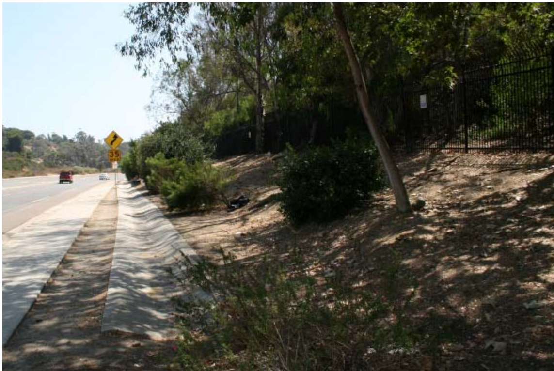
Figure 22. Site 14 - Gate Entrance - South
