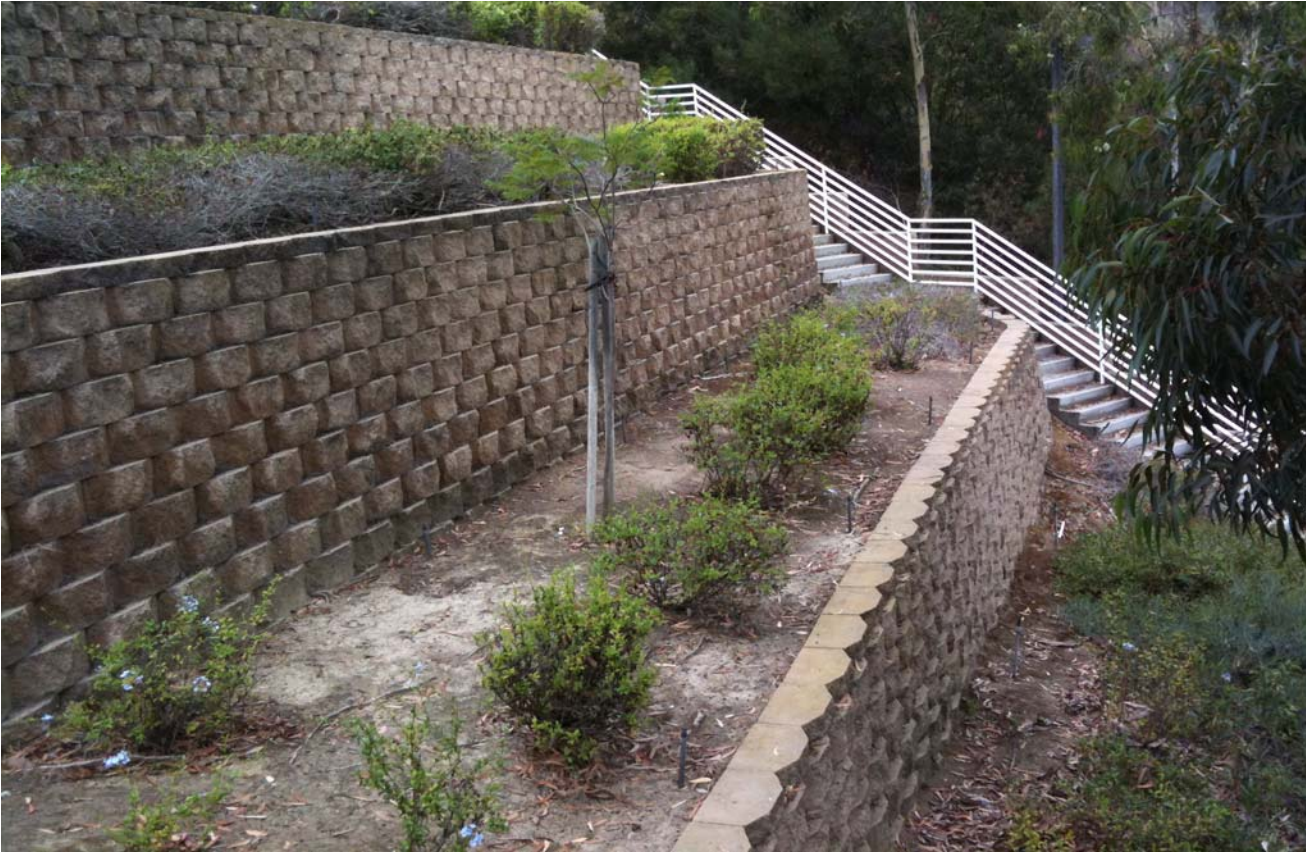
Photo 3-16. Retaining wall below Fischer House.
