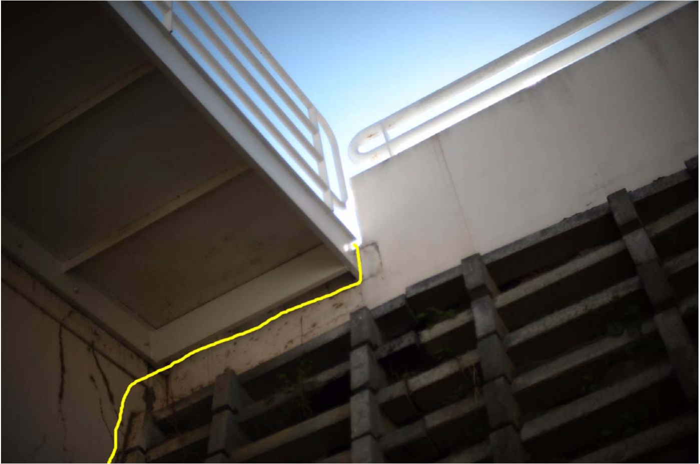
Photo 3-5. Yellow line depicts suggested route of proposed gutter.
