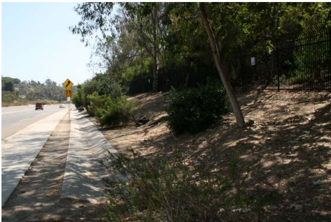
Figure 22. Site 14 - Gate Entrance - South
