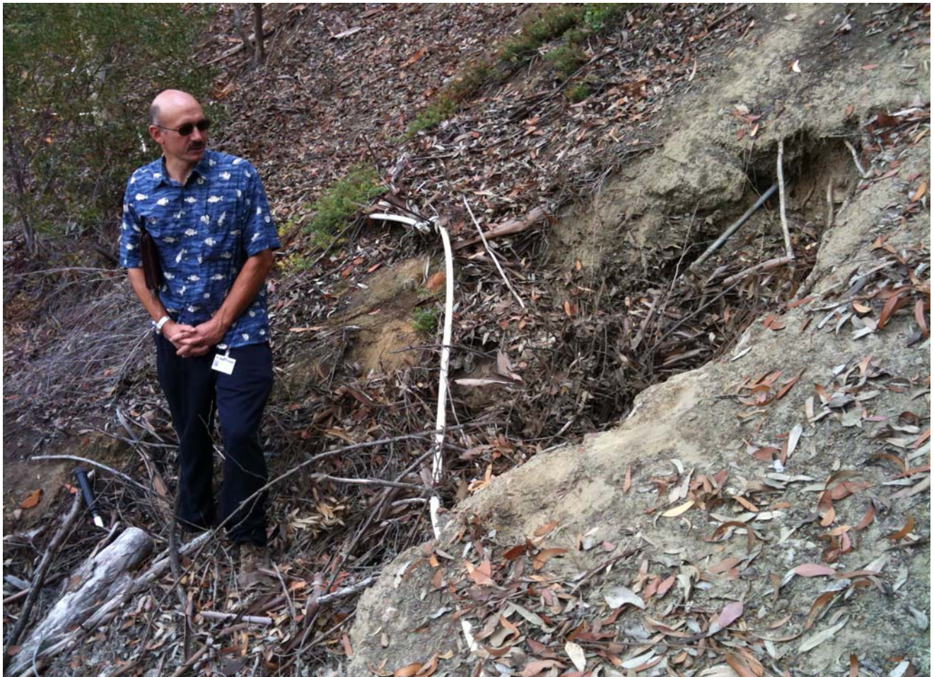
Photo 3-9. Large gully erosion filled with slash. Note irrigation system in disrepair.
