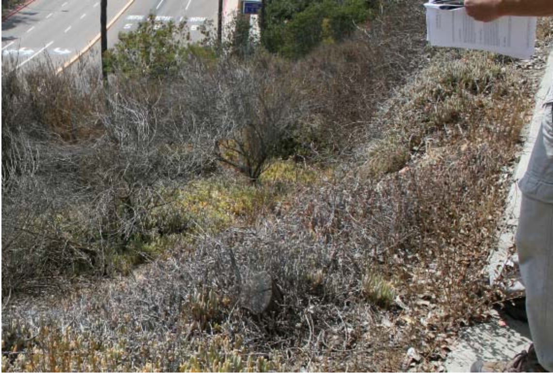
Figure 16. Site 9 - Crib Wall Restoration.
