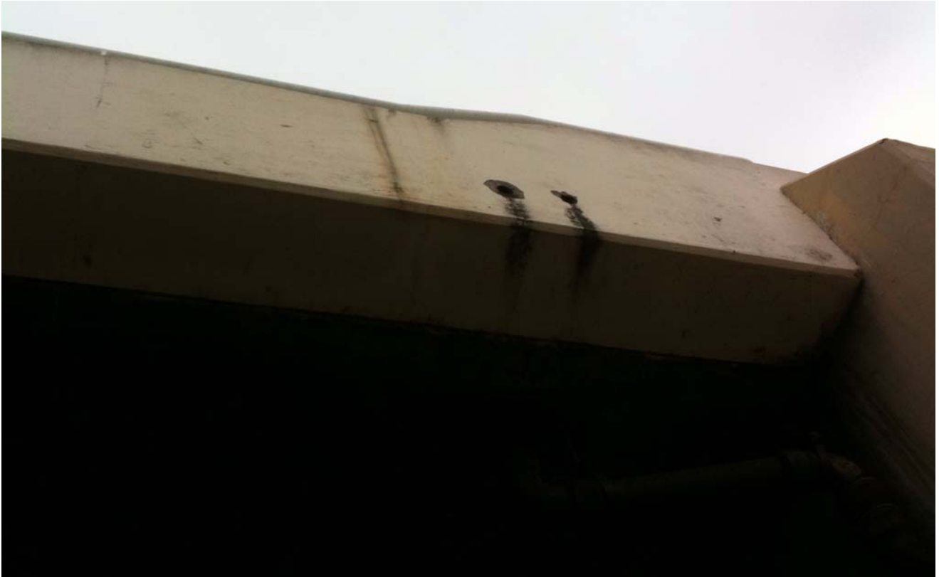
Photo 3-18. Drainage holes in parking structure above that provide the water source.
