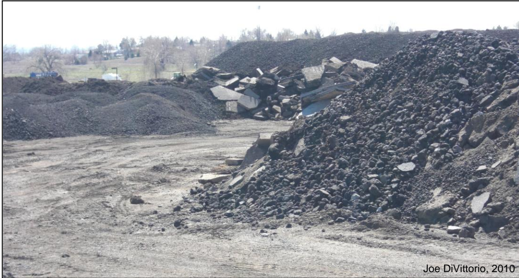
Figure A-2. Fill materials separated by type – soil, broken concrete, pavements, etc. – temporarily stored at a barrow site (photo courtesy of Joe DiVittorio, 2010).
