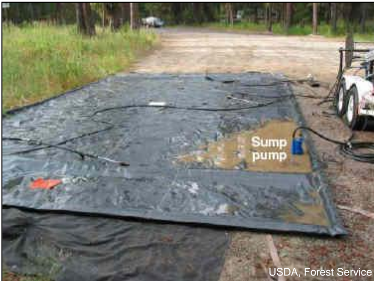
Figure B-1. Bermed portable mat system with sump pump for water recycling (U.S. Department of Agriculture, Forest Service site).
