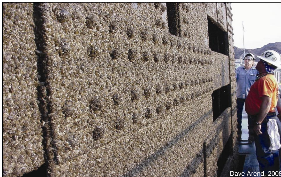
Figure A-11. Mussels covering a penstock gate at Davis Dam (photo courtesy of Dave Arend, 2008).
