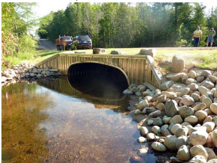
(Above) The West Branch of the Sturgeon River at Lewis Road prior to the culvert replacement project, and (below); The new, bottomless culvert that will allow for uninhibited aquatic organism passage along with reducing sedimentation and thermal pollution.
