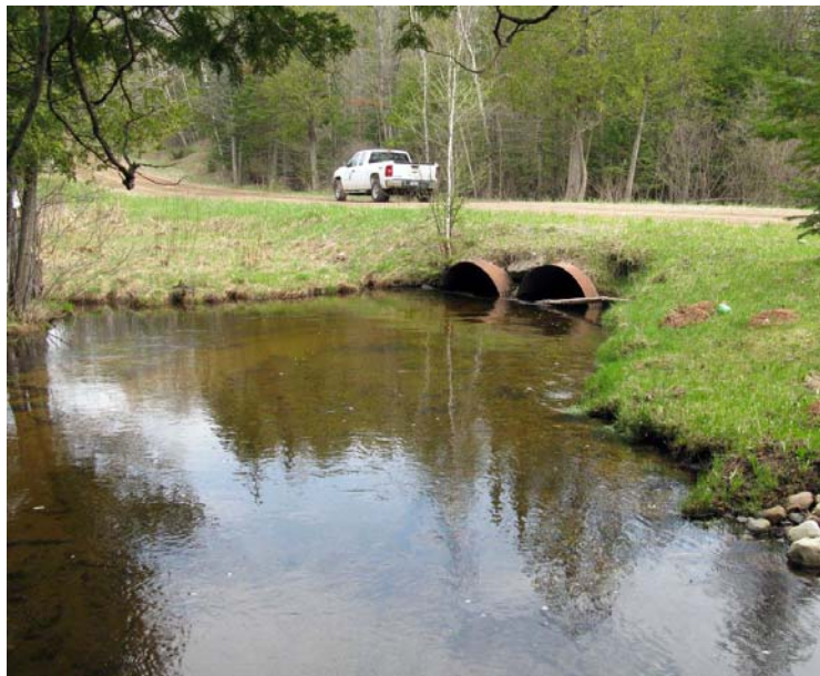
(Above) The West Branch of the Sturgeon River at Lewis Road prior to the culvert replacement project, and (below); The new, bottomless culvert that will allow for uninhibited aquatic organism passage along with reducing sedimentation and thermal pollution.
