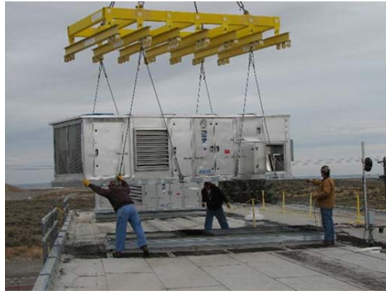
HVAC Replacement at 2750E Building
