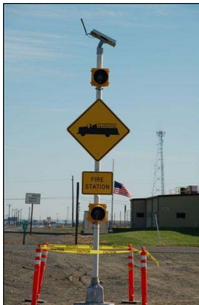
Recently installed Fire Station Warning Signal on Route 3 Eastbound
