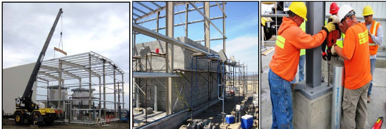
Construction Activities at Sewer Lagoon in 200 West Area
