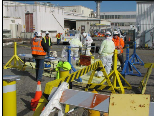
Preparation for disconnecting power cables at 329 Building
