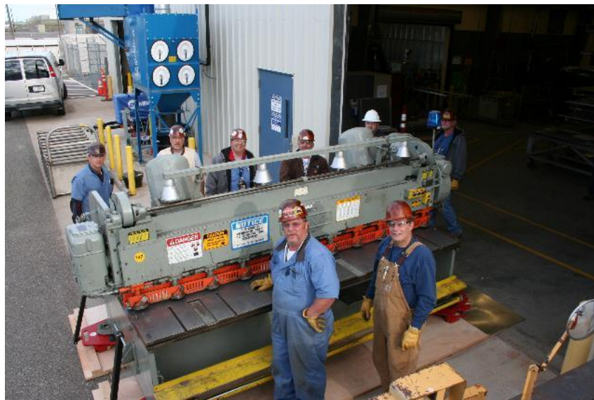
Old shear removed from 2266/200E.
