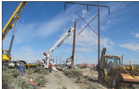
Riggers replacing 75-foot electrical poles
