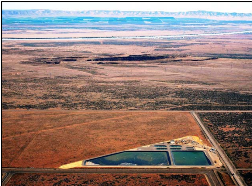
Aerial view of the Lagoon Complex looking north
