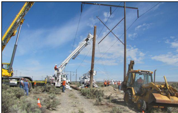
Riggers replacing 75-foot electrical poles
