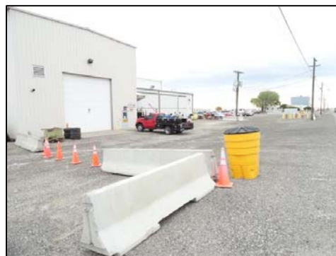
Jersey barriers at 2711E Facility
