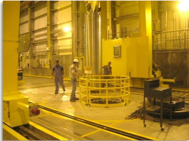
The first Multi-Canister Overpack container of Knock-Out Pot sludge is offloaded at the Canister Storage Building
