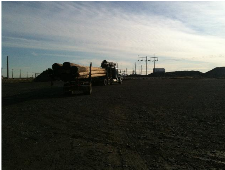
Transmission Poles Arrive on Site
