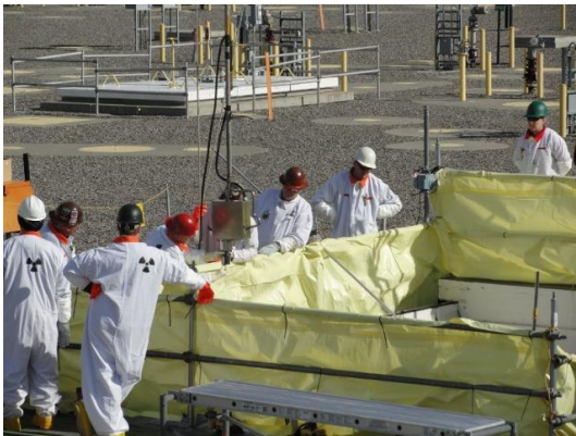
AP Farm installing spacers on jumpers B
