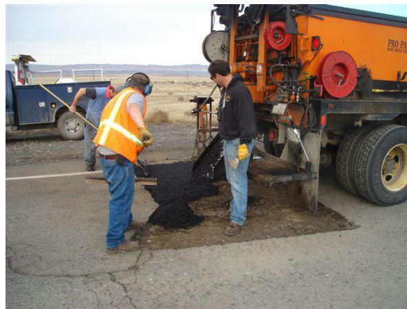
Road Crews work on repairing Route 6.
