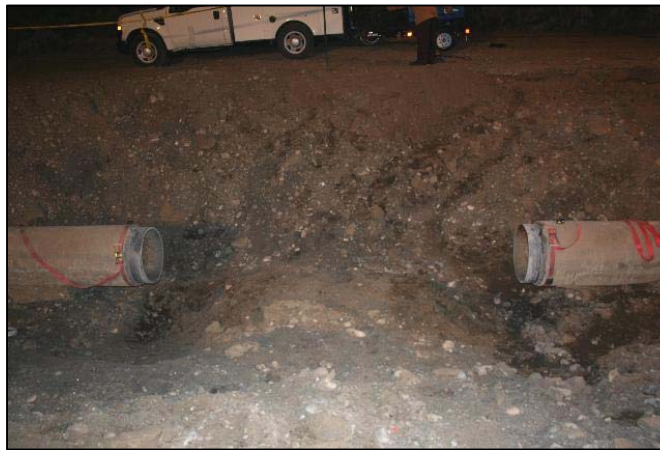
Emergency repair of the leaking export water main
