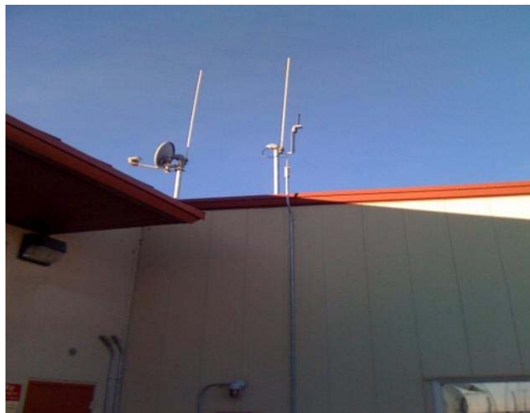
New Warning Signal Antenna Installed on 609A Fire Station
