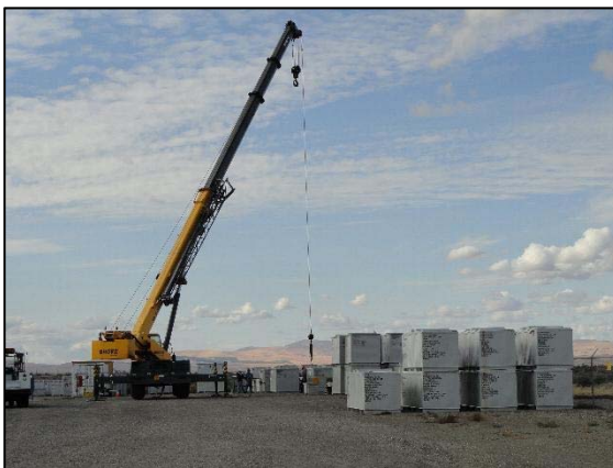
Crane & Rigging Services performing weight and measure activities of burial boxes
