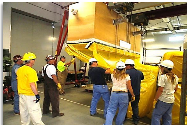
Workers use a mockup to prepare for the disposition of a large glovebox.
