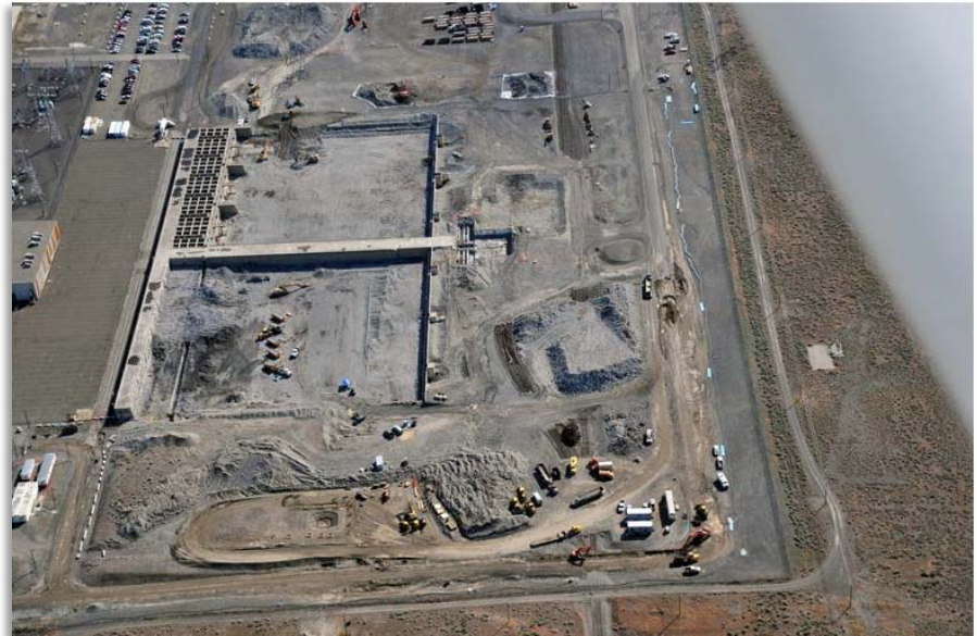
183KW Complex - Demolition Areas
