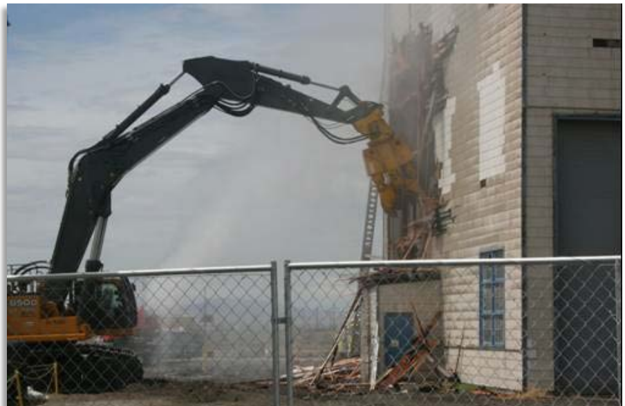
Demolition of 272E Building
