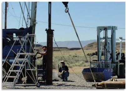
A drilling crew installs a monitoring well in the 100-BC-5 area, where CHPRC will install a total of six wells with Recovery Act funding to support characterization and removal of chromium contamination in the groundwater
