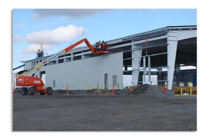
General contractor Skanska USA Build Inc. installs siding on the Radiological Building that will be one of two main process buildings for the 200 West Groundwater Treatment Facility.
