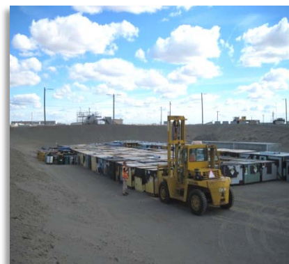
Container Receipt and Placement
