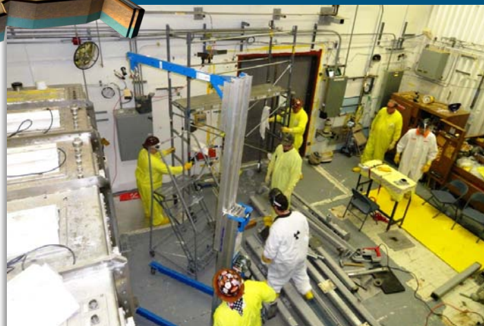
Room 230C Removing Seismic Structure around HC-230C-3.
