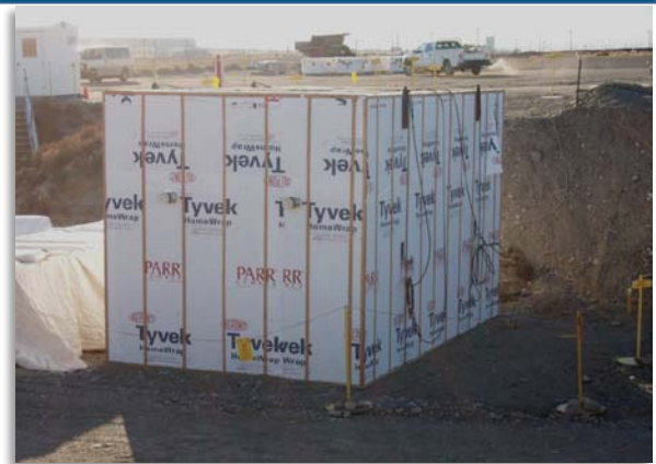
3A Trench 17 Box 80 with Temporary Wooden Cover Installed
