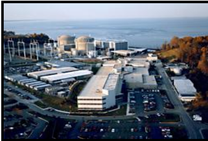
Figure 3: Calvert Cliffs Nuclear Power Plant Source: NRC
