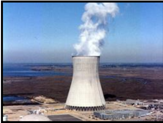
Figure 6. Hope Creek Nuclear Power Plant Source: NRC
