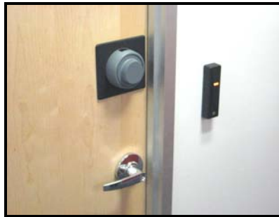
Figure 1. File Room Entrance Secured
