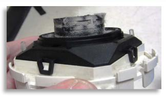
Regular inspections of fire detection and alarm systems are intended to find and correct problems like this dust accumulation that could affect detector performance. *Photo courtesy of Byron Blake.*
