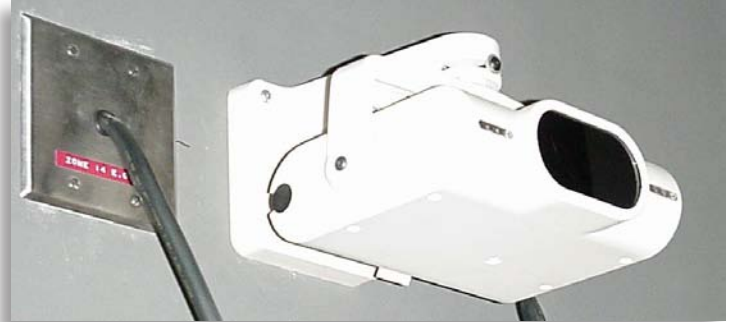
This beam detector transmitter is listed for open area protection.
