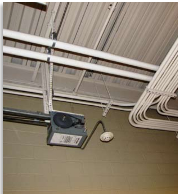
The placement of this spot-type detector should be evaluated by the code official to assess its potential performance.
