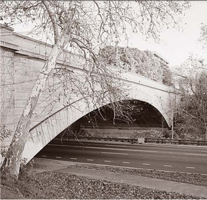
Parkway Bridge Image
