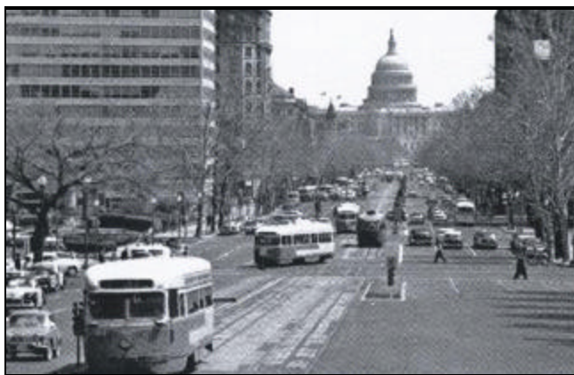
Figure 5 – Historical photo* of Pennsylvania Avenue with streetcars in the middle of the street in 1959
