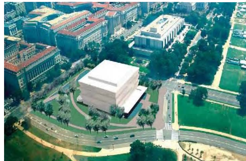
Figure 3.3.31 Refined Pavilion Alternative: View from the Top of the Washington Monument Looking Northeast
